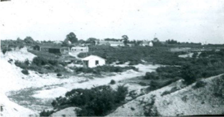
View looking north across the gravel workings - Bakers Lane houses in the distance 1947 Alf Fisk
