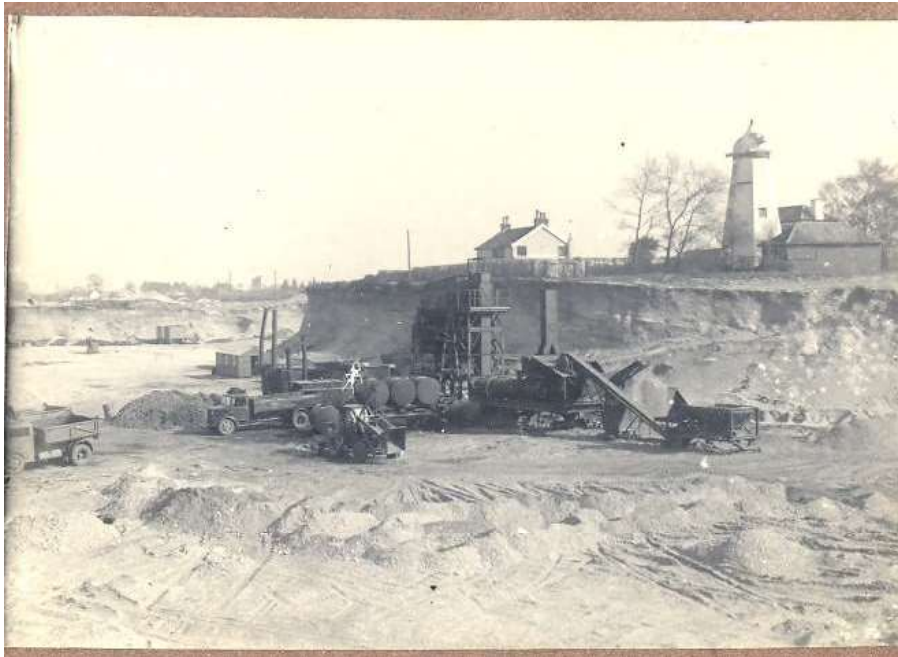
Loading the gravel from the cliff below the Mill, approx 1940's. Alf Fisk
