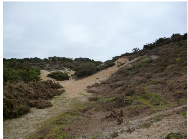
After clearance (showing cut material)
