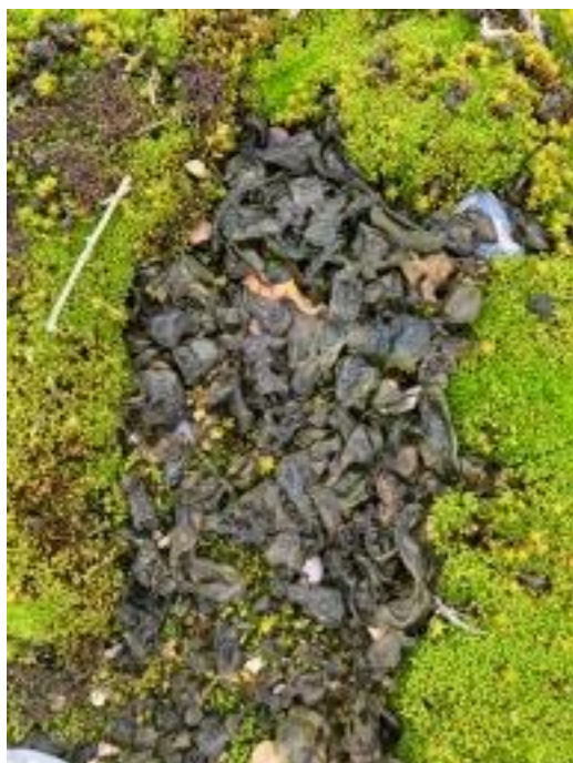
Nostoc (a photosynthetic bacterium) on the concrete square.
